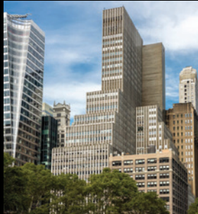
5 BRYANT PARK MAJOR LOBBY RENOVATION COMPLETE
