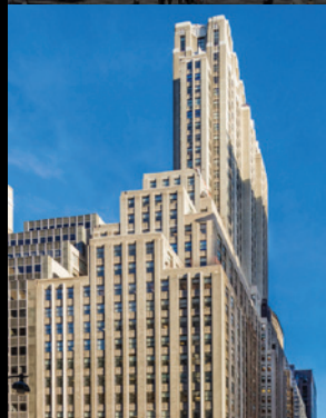
521 FIFTH MAJOR LOBBY AND BUILDING RENOVATION UNDERWAY
